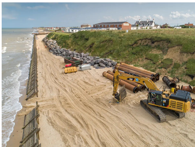
This picture is from an area of the Norfolk coastline near Bacton which is being protected from erosion by the creation of artificial sand dunes .
